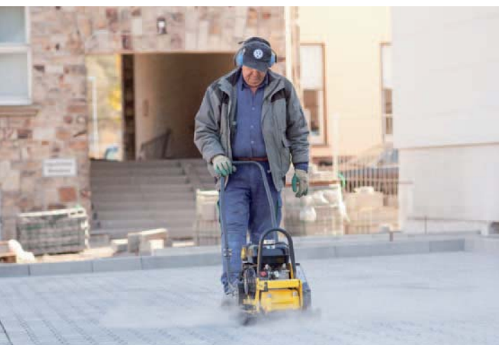
...and block paving.
